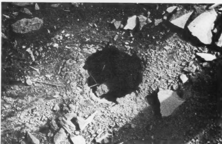
Seven-inch crater in stonemasonry floor outside embassy entrance marks impact of terrorist bomb. It blew out 115 large windows on front side of building.
